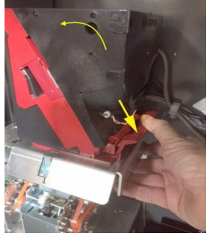
Removing a Mini-hopper
